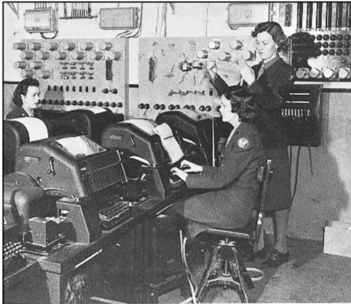
WACs assigned to the Eighth Air Force in England operate teletype machines. (DOD photograph)
